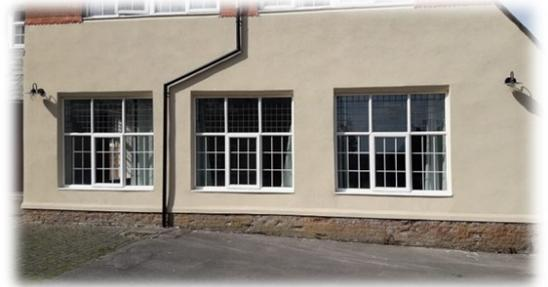
cay, but it had trapped the moisture in the wall, which led to the rusting of the steel reinforcement in the window heads, decimating their strength.
